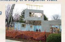
**Stronger.** Superior Walls precast concrete wall panels are constructed for use below or above grade. They are ideal for any residential or light-commercial construction. Superior Walls AG Systems are designed to be used in conjunction with our
